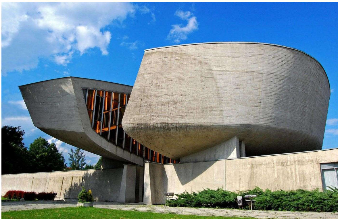
Museum of the Slovak National Uprising in Banská Bystrica (MSNU)
